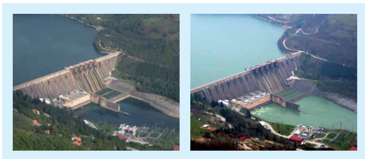
Figure 37: Spot the difference? The Bajina Bašta plant in Serbia was upgraded in the five years 2008-2012 from 4x 95.4 MW turbines to 4x 105.6 MW, increasing output by 13% (=40 GWh additional generation per year) without changing the plant's appearance.
