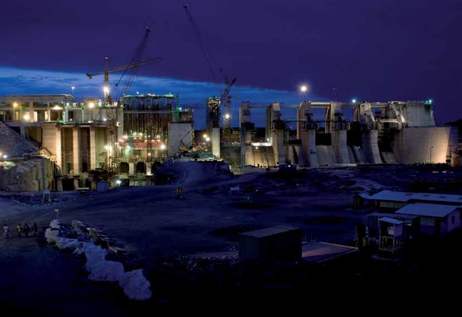
Construction of São Salvador hydropower plant, Brazil.
