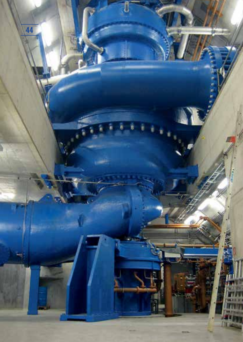
Figure 33: The Kops II multi-stage ternary pump-turbine (Austria)
