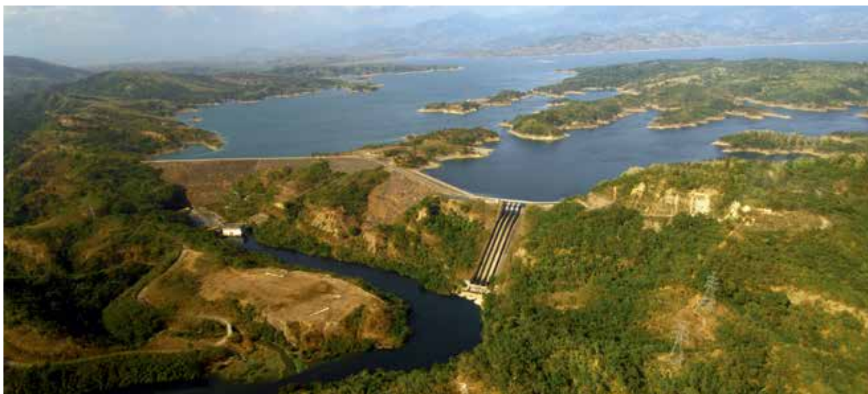
Pantabangan lake, Philippines, showing dam, spillways and power station.
