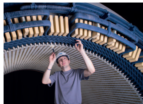
□ Inspection du stator
