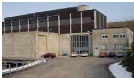
▣ Bjurfors Nedre hydropower plant
