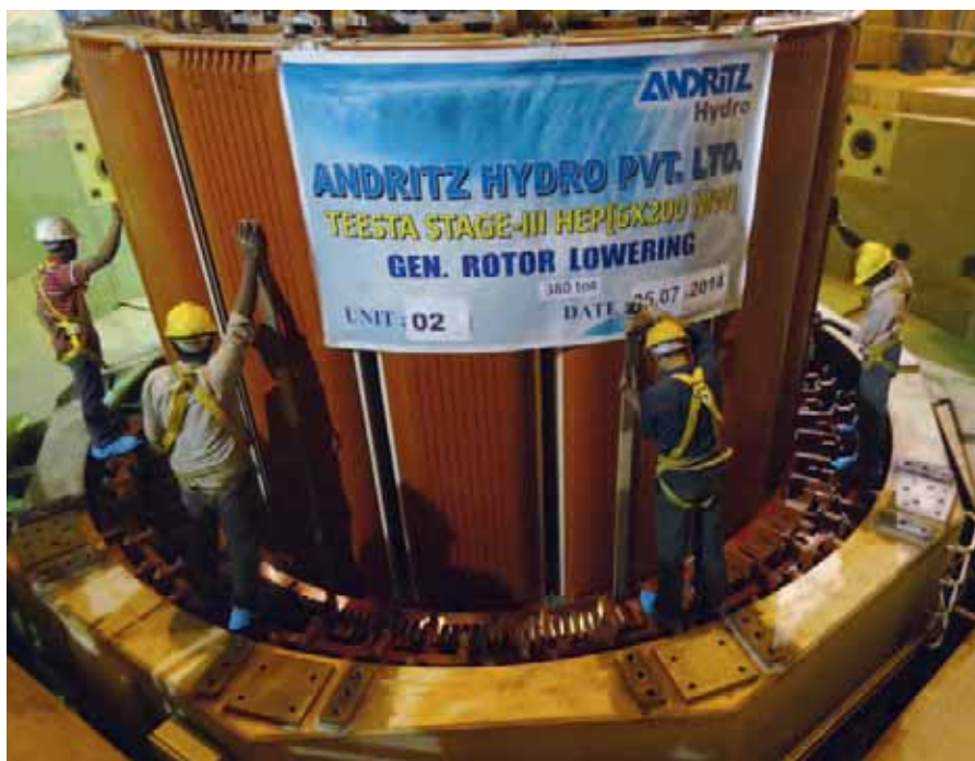
Rotor lowering in unit #2
