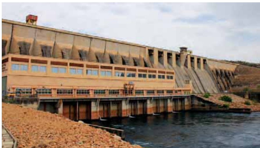
Hydropower plant and spillway
