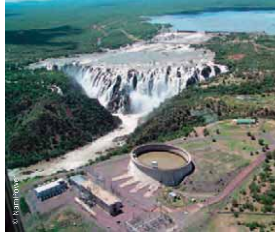
□ Aerial view on Ruacana hydropower plant
