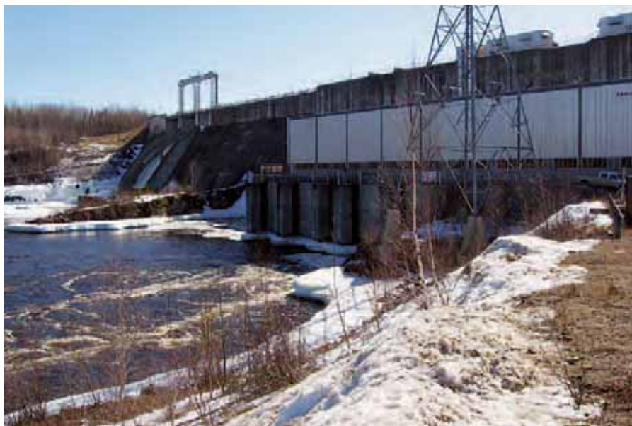
▼ Lower Mattagami hydropower plant
