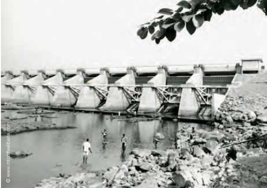
□ Mount Coffee Dam in its original condition
