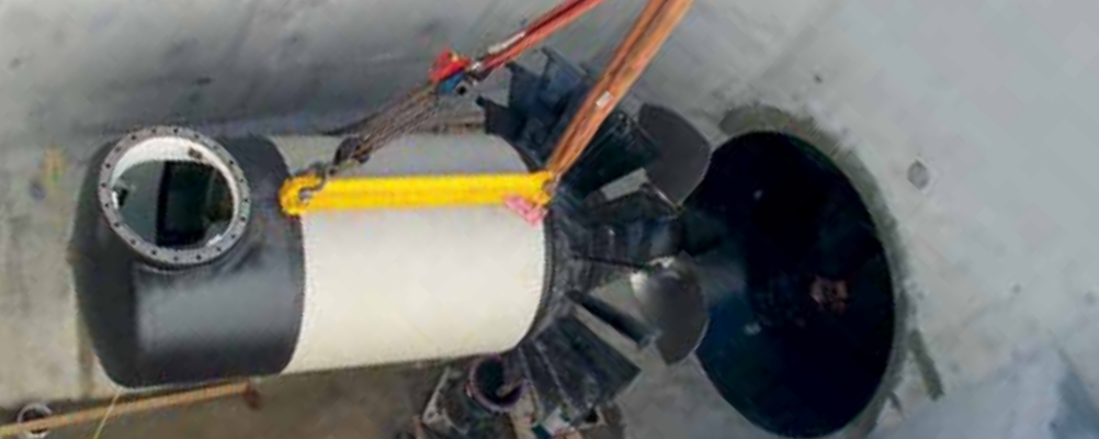
▣ ECOBulb™ lifting into powerhouse
