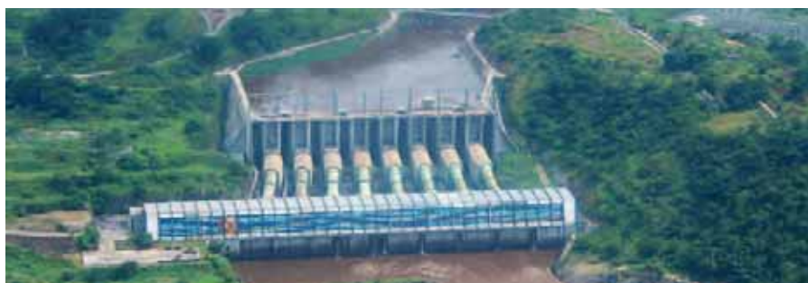
Aerial view of Inga 2 hydropower plant
