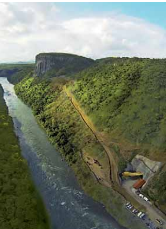
▣ Kwanza River and future power house access of HPP Laúca
