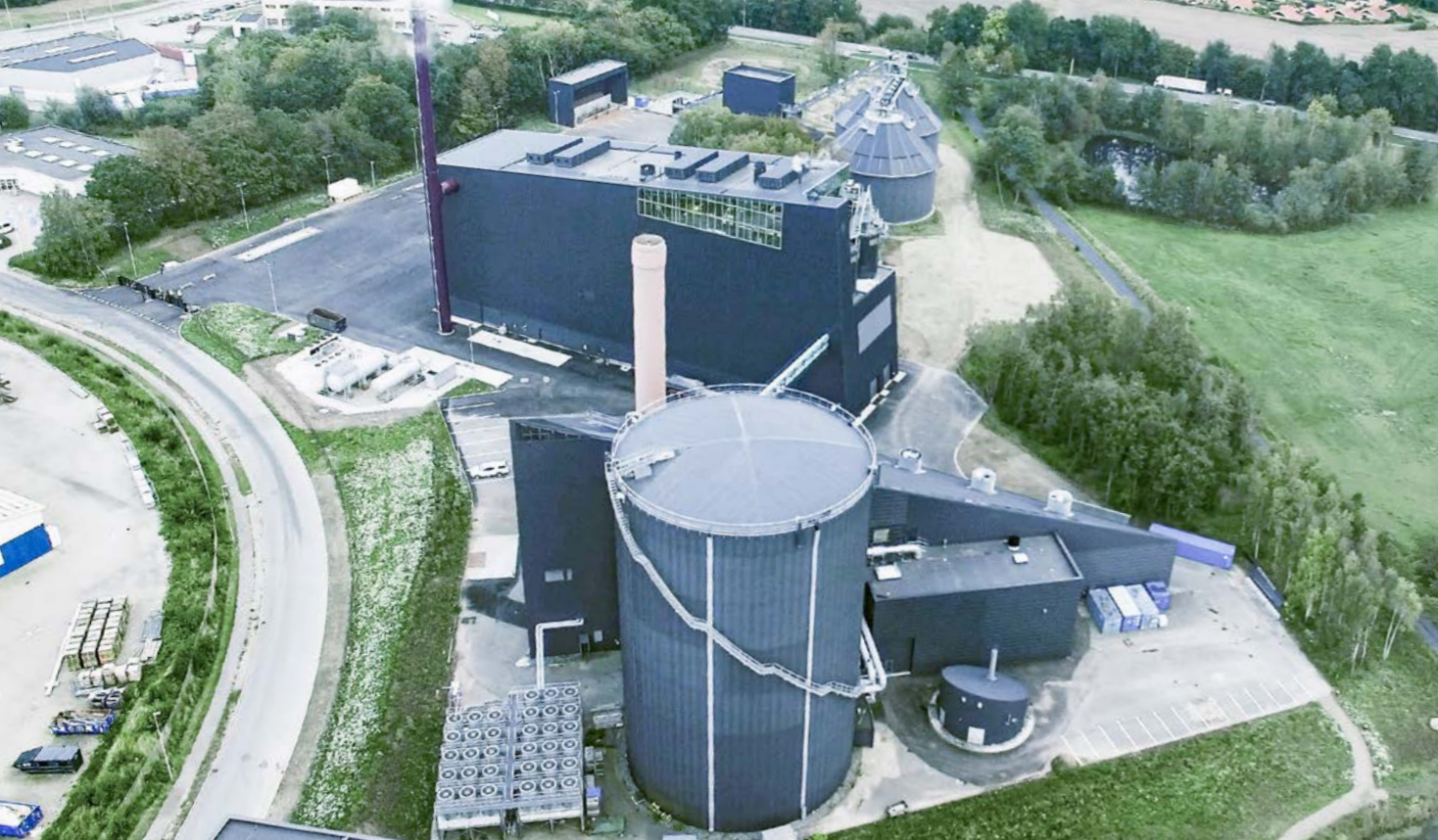
ANDRITZ's scope of supply included the boiler island, from fuel silos to boiler outlet, based on its Ecofluid BFB boiler design.
