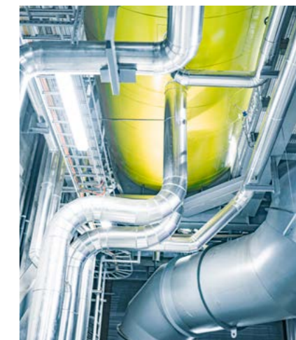
The plant is now fully operational and ready for its first winter of operation.
