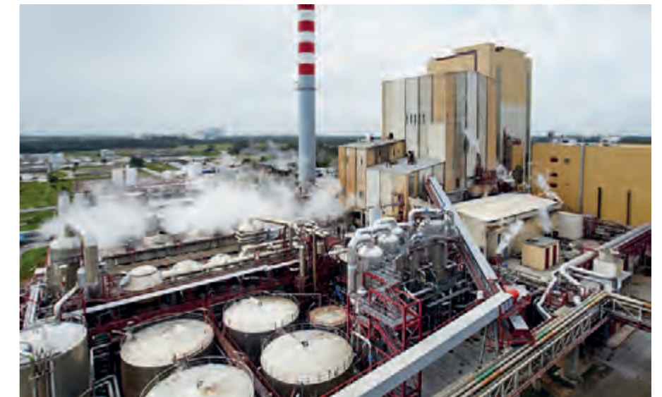
▲ New four-effect evaporation plant shown in foreground. ANDRITZ recovery boiler (installed in 2005) in background.
