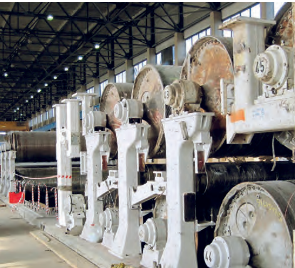
▲ ANDRITZ has developed detailed procedures for relocating paper machines and has the capability to modernize or upgrade the machine before reinstalling it.
