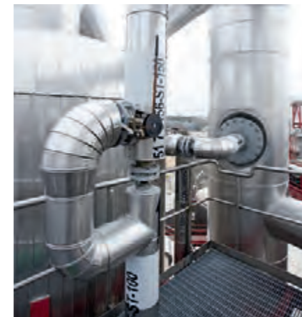
▲ Duct stripping technology (patented technology from ANDRITZ) which removes methanol and residual sulphur components from condensate flows. The benefits are significantly reduced COD to the effluent treatment plant, less energy usage when heating secondary condensate, and lower water consumption by using clean odorless condensate instead of fresh water.
